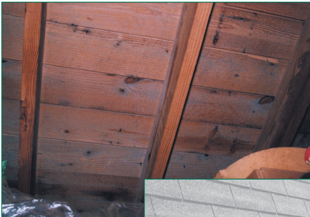
Figure 6—Mold/mildew in a humid southern climate. While attic insulation was properly held back at the edge and openings were present in the soffit cladding, the eaves carpentry was continuous along the entire perimeter. The mold/mildew colonies were fostered during a wintertime condensation scenario, drying to the powder during the hot season as shown.
