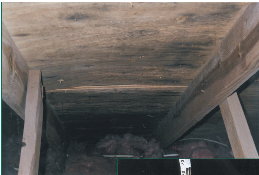
Figure 2—Moisture will accumulate in a wood deck long before water droplets are formed. Note the buckled plywood deck, mold formation, and soffit region blocked with glass fiber insulation
