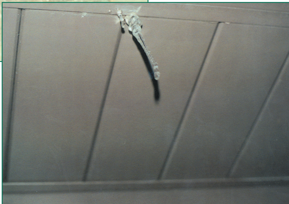
Figure 1A and 1B (below)—Ice damming on a roof where ice and water membrane was not provided.
