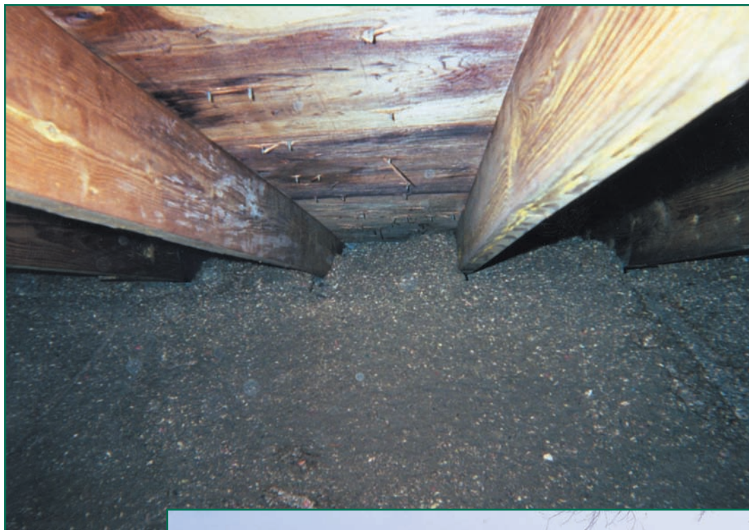
Figure 4—Attic insulation must be held back from the soffit region in order to serve as the intake port. A pre-manufactured baffle can be used to keep blown-in insulation from becoming a ventilation impediment.
