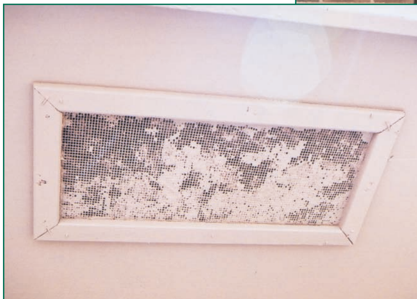
Figures 5a and 5b—Multiple coats of paint can render soffit openings virtually useless. Airways and vent openings should be slightly larger than would be implied in the sizing calculation.
