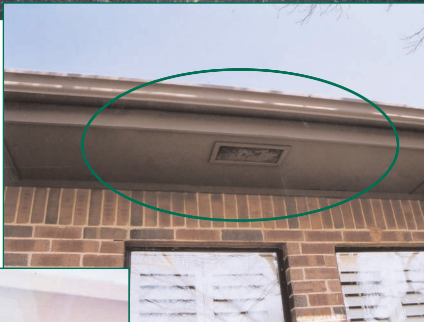
Figures 5a and 5b—Multiple coats of paint can render soffit openings virtually useless. Airways and vent openings should be slightly larger than would be implied in the sizing calculation.
