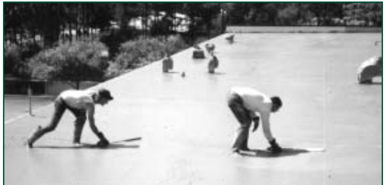
If applied correctly, lightweight insulating concrete is one of the best wind uplift performers available. (Photo by Celcore Inc.)
