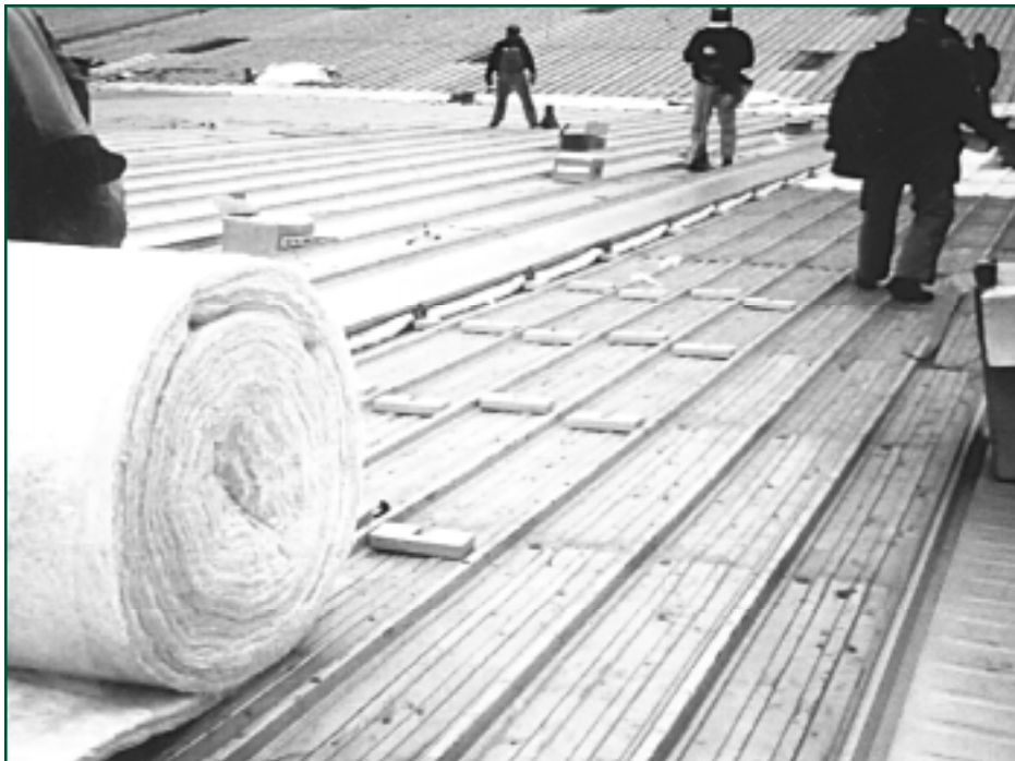
Figure 20 — This standing seam metal retrofit system utilizes a standing seam roof clip attached directly to the underlying structural member.
