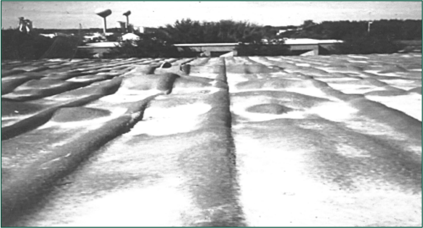
Figure 15 — The through-fastened R-panel rib pattern through the applied foam.
