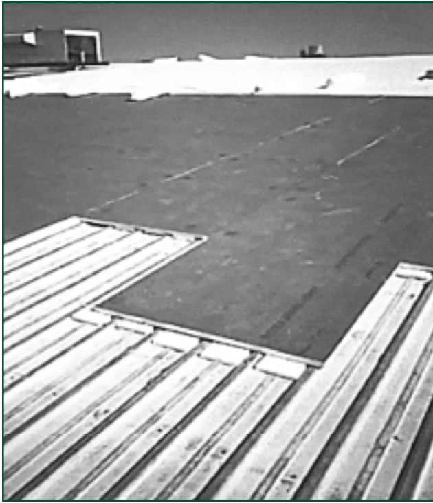
Figures 16 and 17 show a 26-gage through-fastened metal roof with a two-layer insulation system and a single ply membrane roof system.
