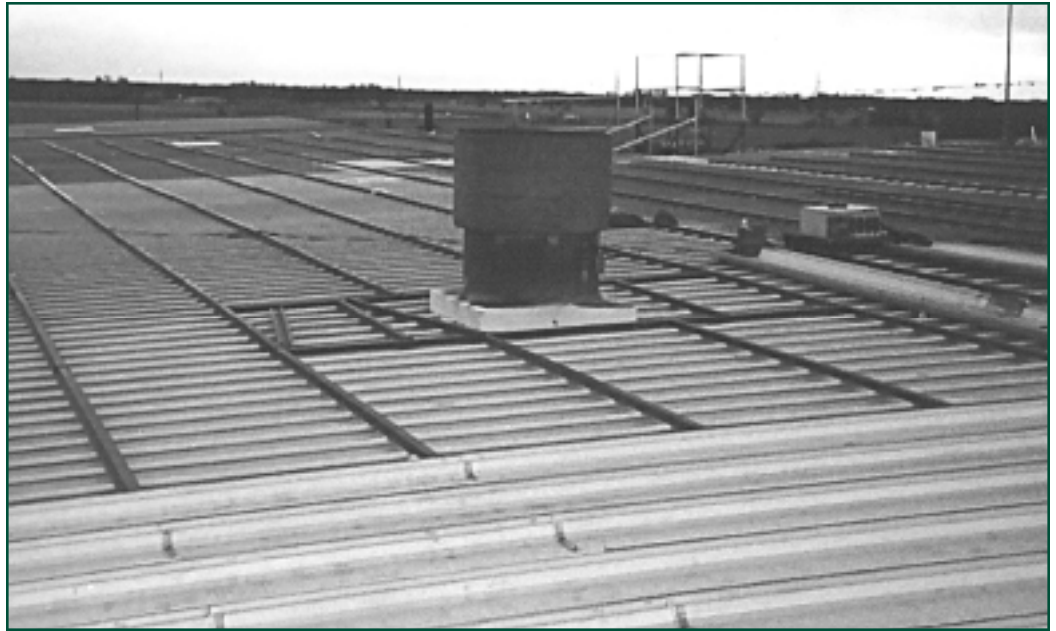
Figure 19 — 16-gage structural members in place directly over the underlying structural members.
