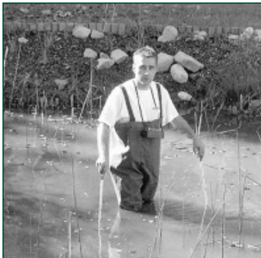
Figure 4: Locating leaks in a geo-membrane liner with the EFVM technique.
