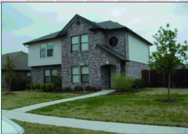
Figure 1: This otherwise attractive building had to be evacuated because of hazardous spores inside caused by inadequate or missing flashing of the masonry veneer. Photo courtesy Norm L. Cooper, P.E.
