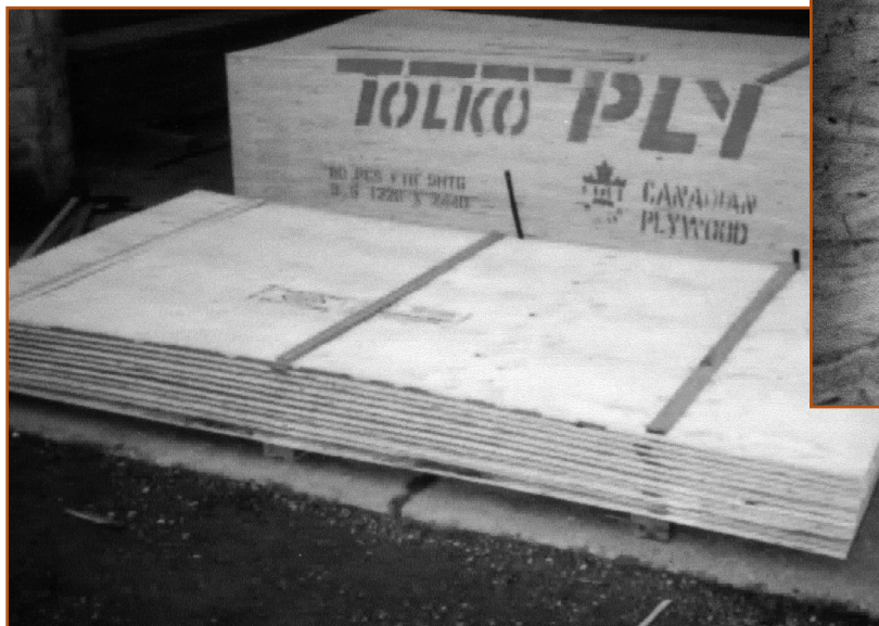
Photo 3: "Stickering" helps to pre-condition the sheathing prior to application.
