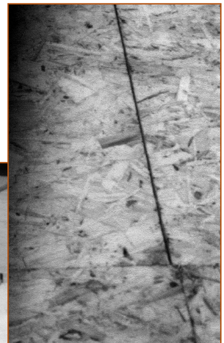
Above: Photo 4: OSB panels are customarily spaced with the shank of a nail.
