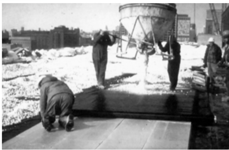
Extruded polystyrene insulation is used in protected membrane roof assemblies.
