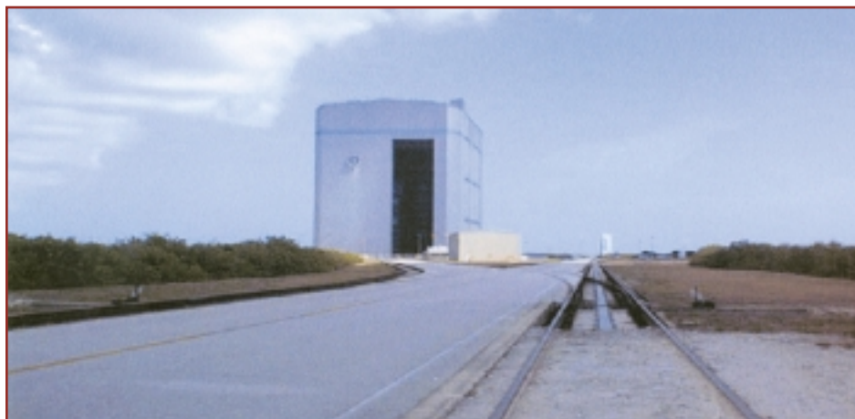
Photo 1: Exterior view of SMARF Building.
