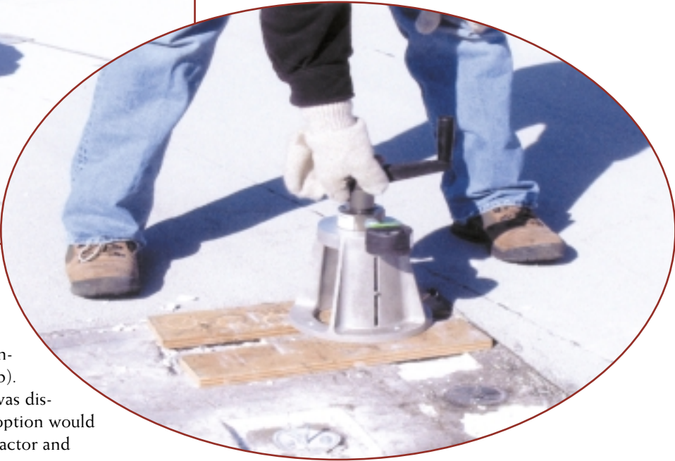
Below: Photo 17: Plywood panels placed on surface to distribute load during testing. Values ranged from 528 pounds to 1,274 pounds. Fasteners are spaced at approximately 1'-0" on centers.
