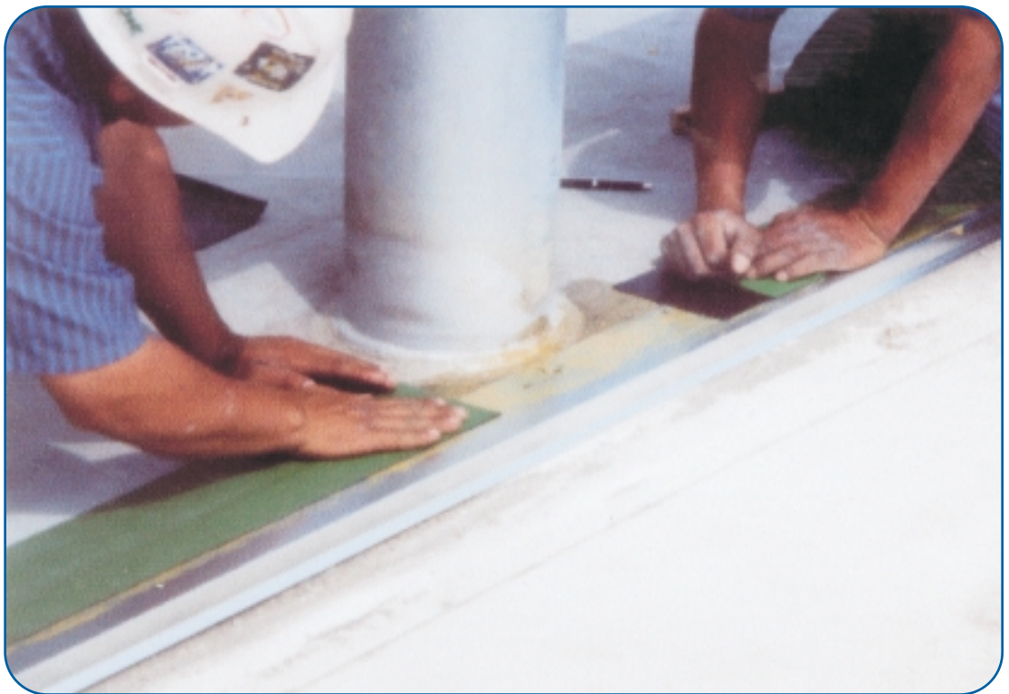
Photo 4: Pre-treatment of cracks on slab to be waterproofed.
