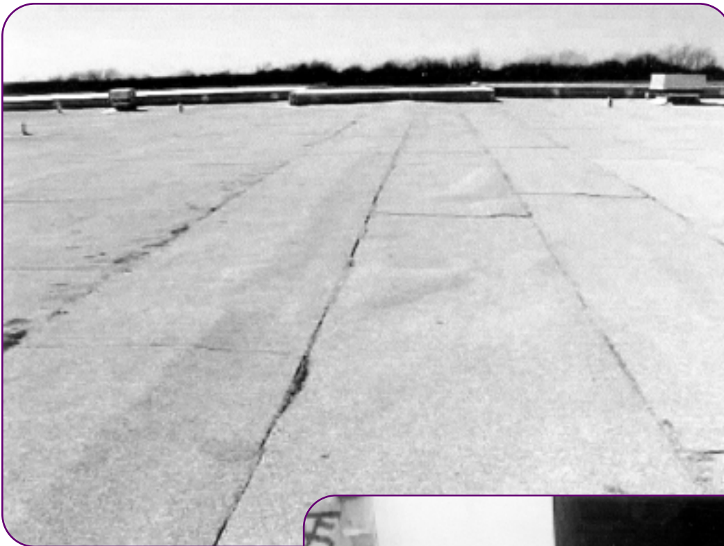
Photo 2: Dual 80 or Bond-Ply assemblies blistered profusely.
