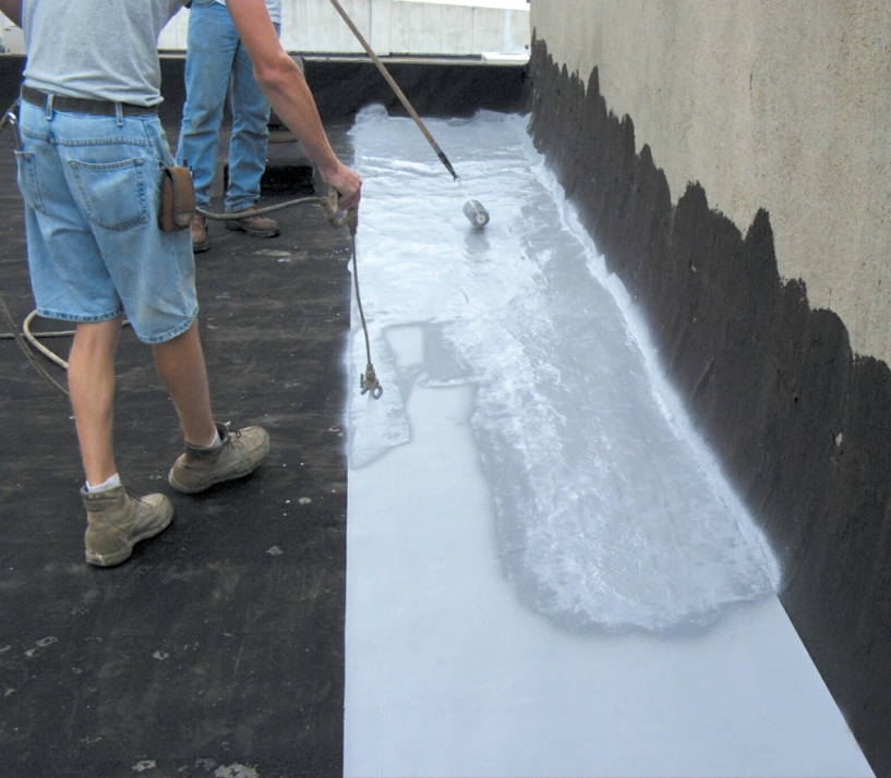
Asphalt restoration with acrylic coatings and foam flashings.
