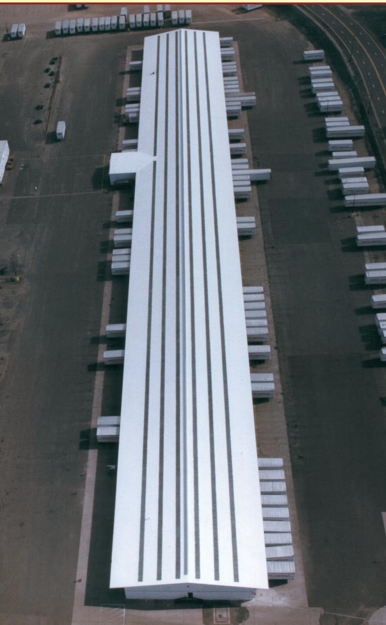
Metal roof restoration.
