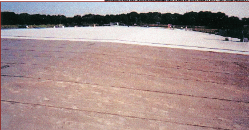
Spray polyurethane foam application over BUR with gravel.
