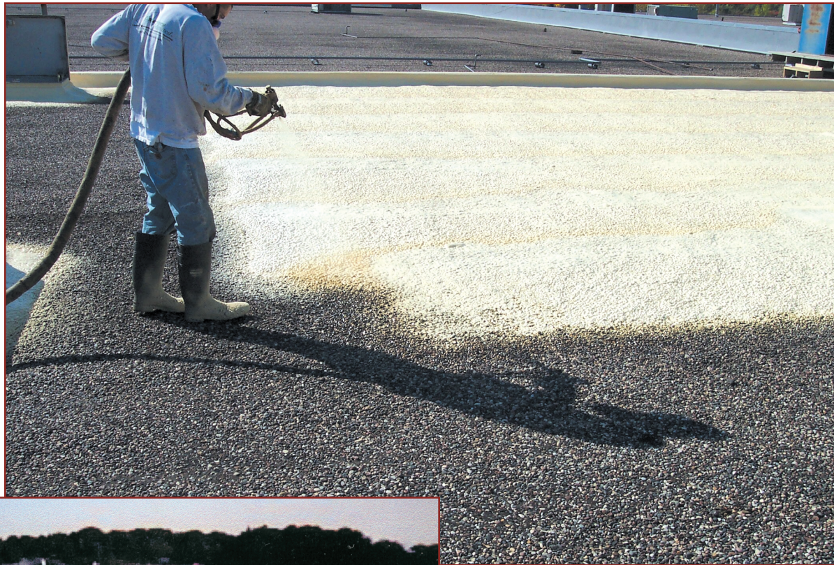
Spray polyurethane foam application over BUR with gravel.
