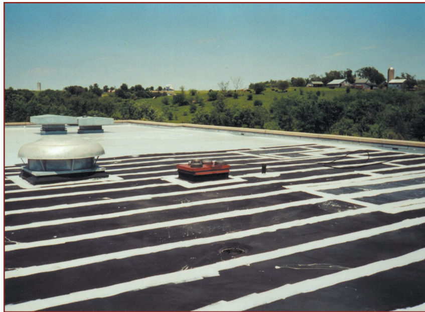
EPDM restoration with seams taped and coated.
