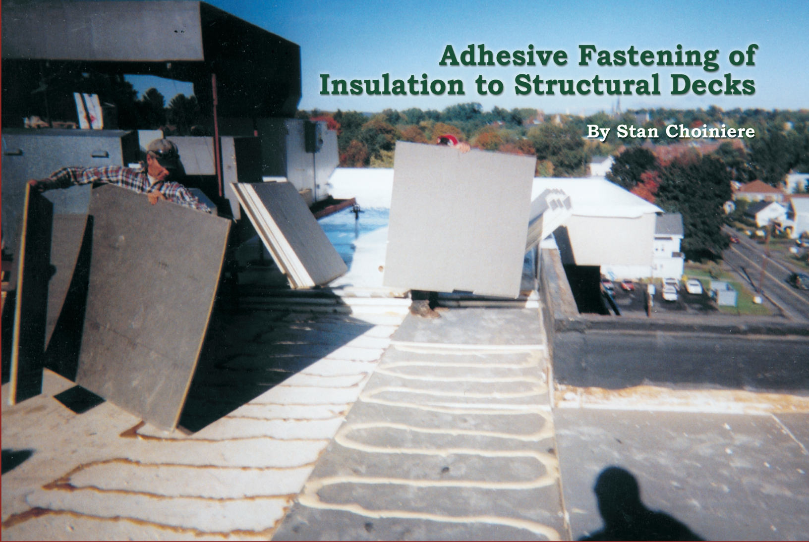
Adhesive applied in a serpentine ribbon form.
