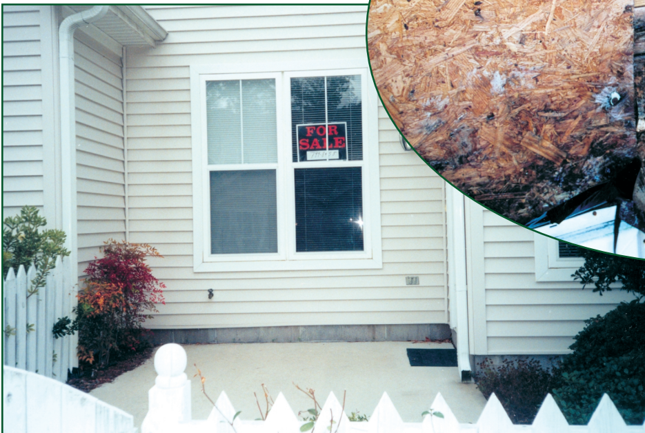
Photos 4 and 5: Views of significant damages below a roof/wall intersection on a building clad with vinyl siding.
