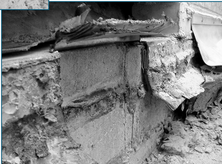
Photo 1 (above) and 2 (right) show roof flashing installed above through-wall flashing
