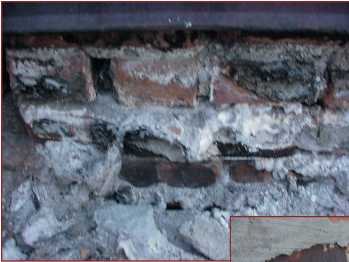
Photos 4 and 5: Moist air condensing behind roof base flashing and deteriorating brick.
