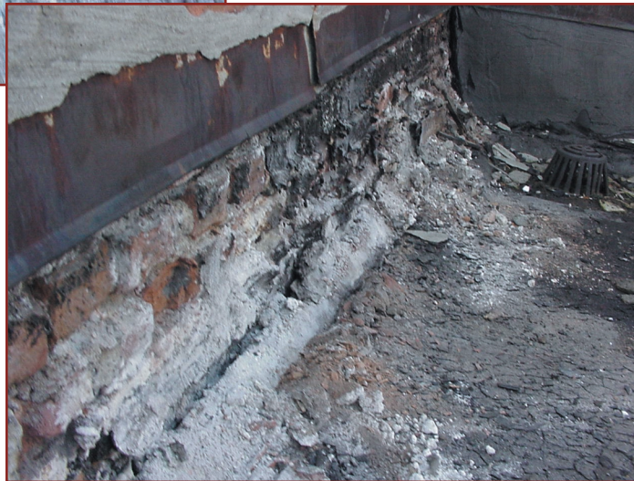
Photos 4 and 5: Moist air condensing behind roof base flashing and deteriorating brick.
