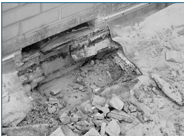
Photo 1 (above) and 2 (right) show roof flashing installed above through-wall flashing
