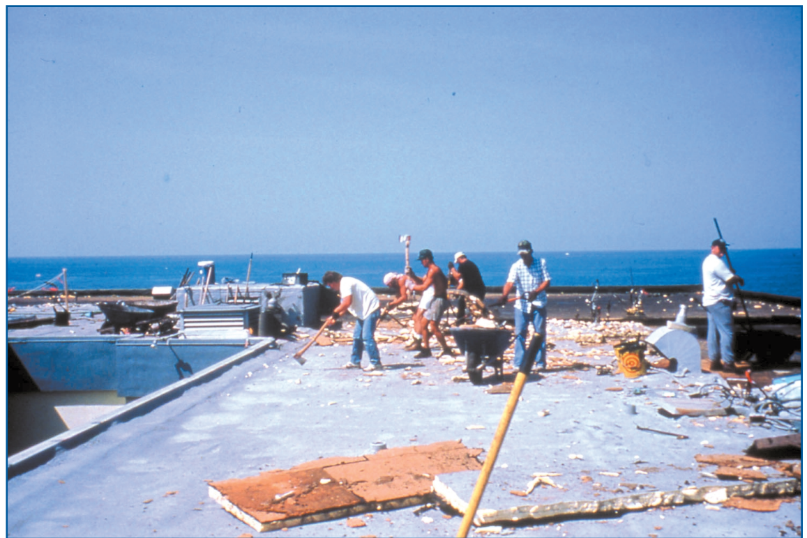
Workers prepare for reroofing after extensive wind damage.
