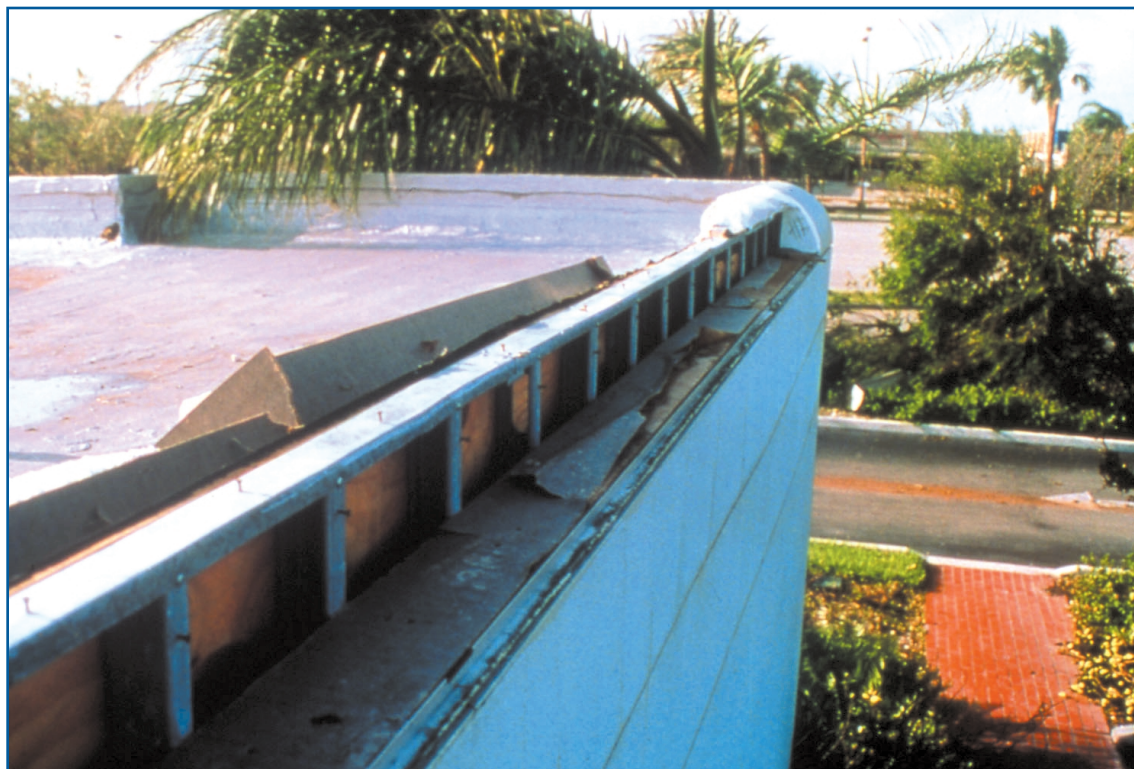
Untested, insecure edge detail.
