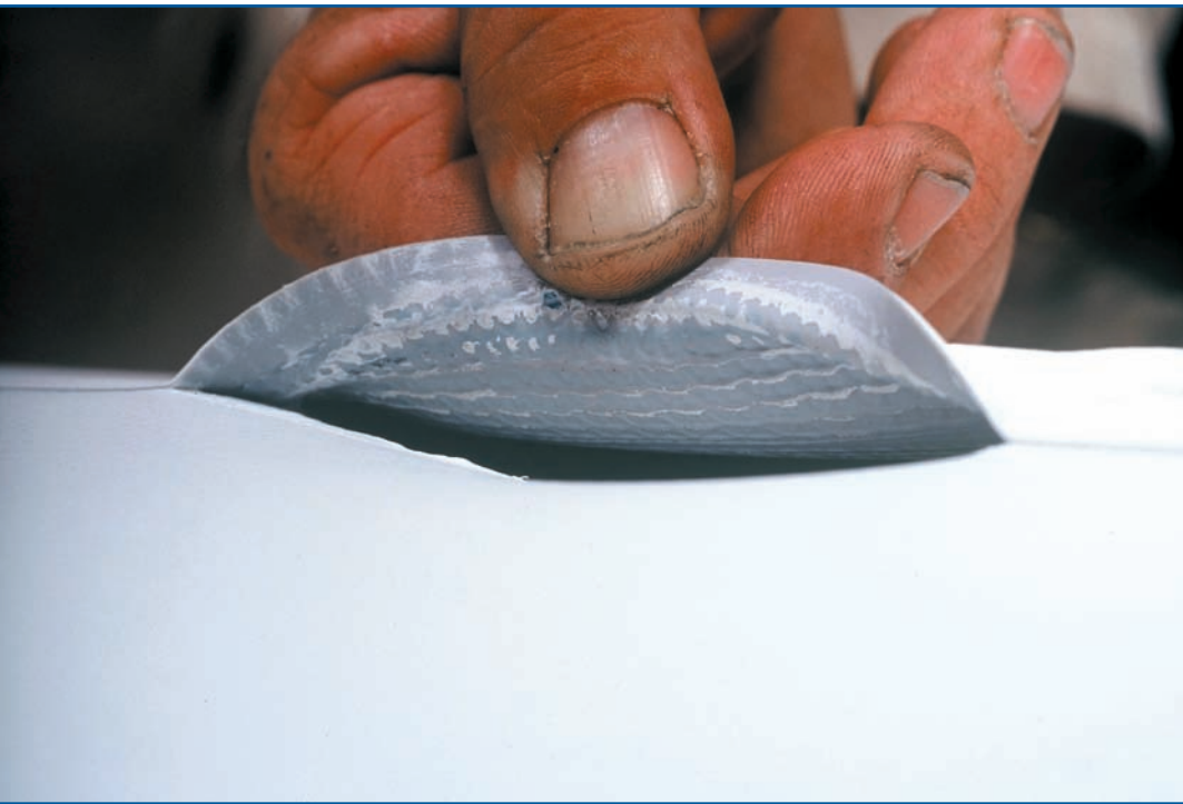
Photo 6: Delamination and membrane tear.
