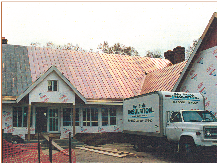
Photo 4: Red lead on a locked and soldered flat-seam, lead-coated copper roof.
