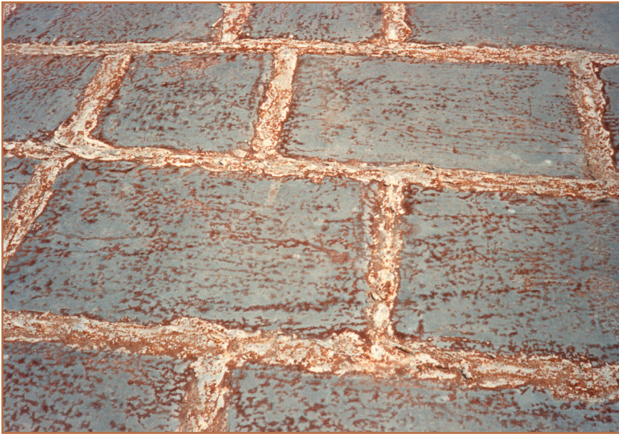
Photo 3: The owner of this roof off the coast of Maine complained that the lead was coming off his lead-coated copper. In actuality, “red lead” patina was forming.
