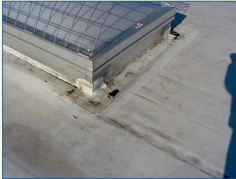
Flashing of a skylight on a thermoplastic roof.
