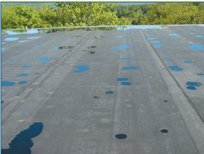
Seams on full-adhered EPDM system.
