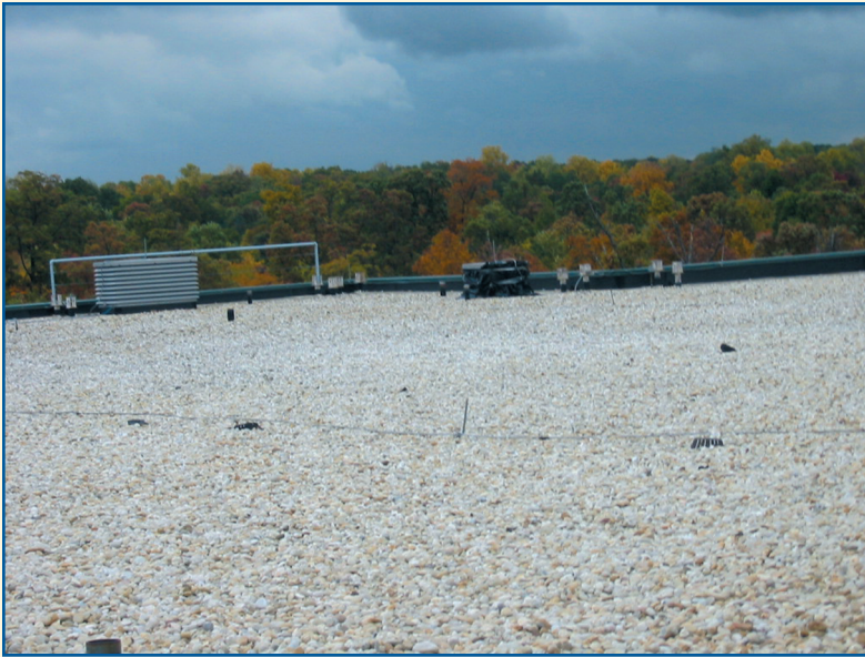
Ballasted EPDM roof.
