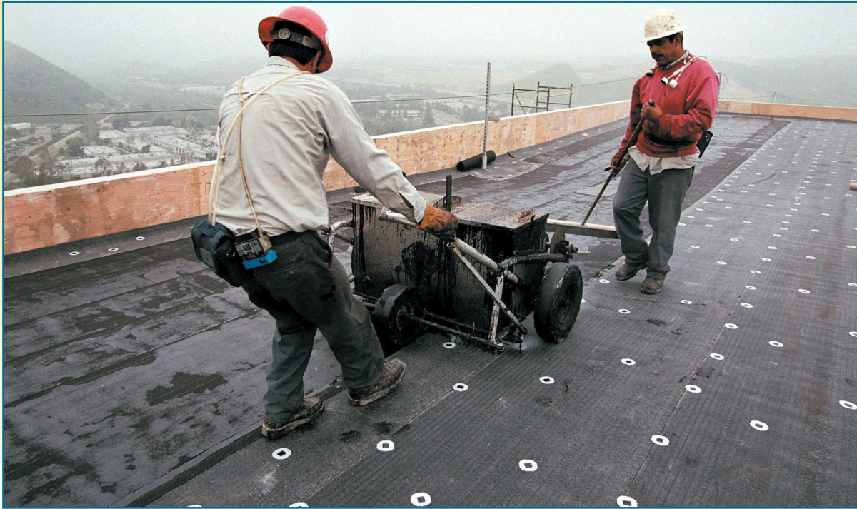
Photo 1: BUR has held a 20 percent or more share of U.S. low-slope roofing sales over the past several years, adding to the 50 billion square feet of BUR in service.
