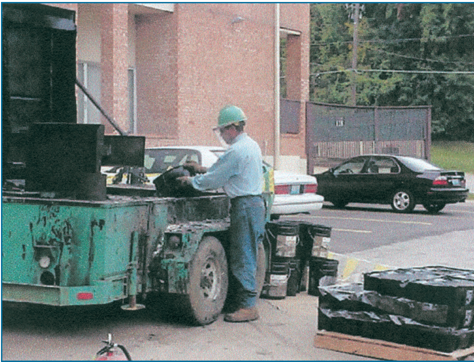
Photo 4: A worker drops a block of low-fuming asphalt into a heating kettle on a BUR job.
