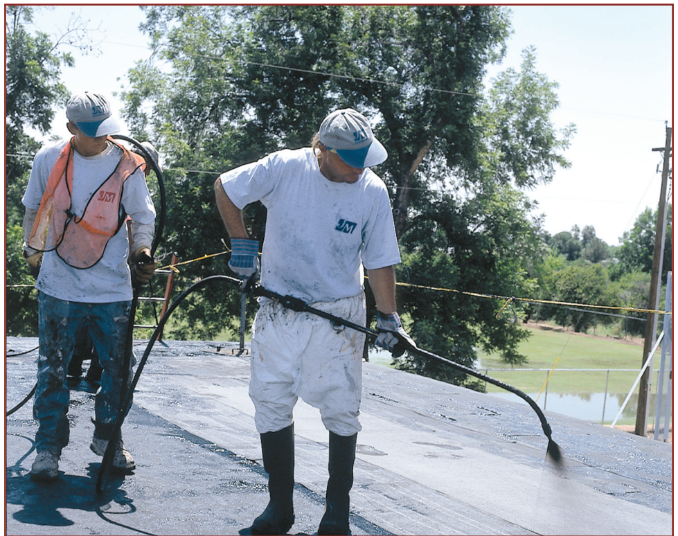
Rofer using spray equipment for a cold application BUR system.
