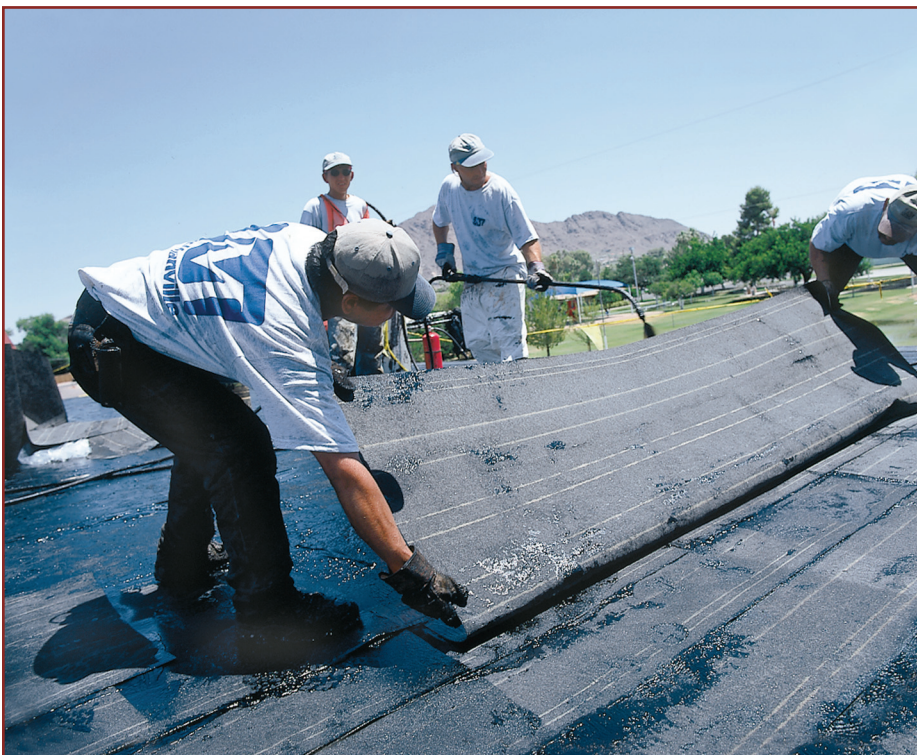
Roofers using the “mop and flop” method with a BUR cold applied job.
