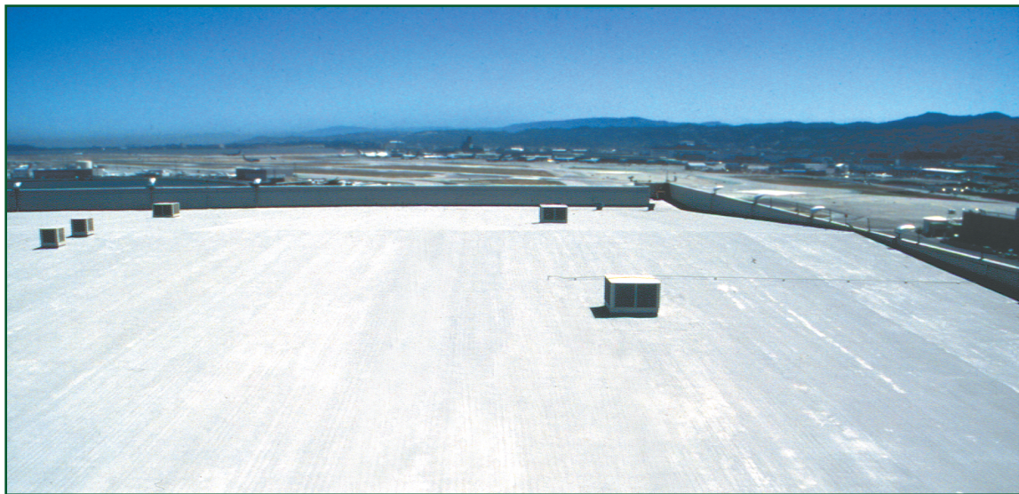
SPF systems are typically coated with light-colored, reflective coatings that utilize the albedo effect to reduce rooftop temperatures.
