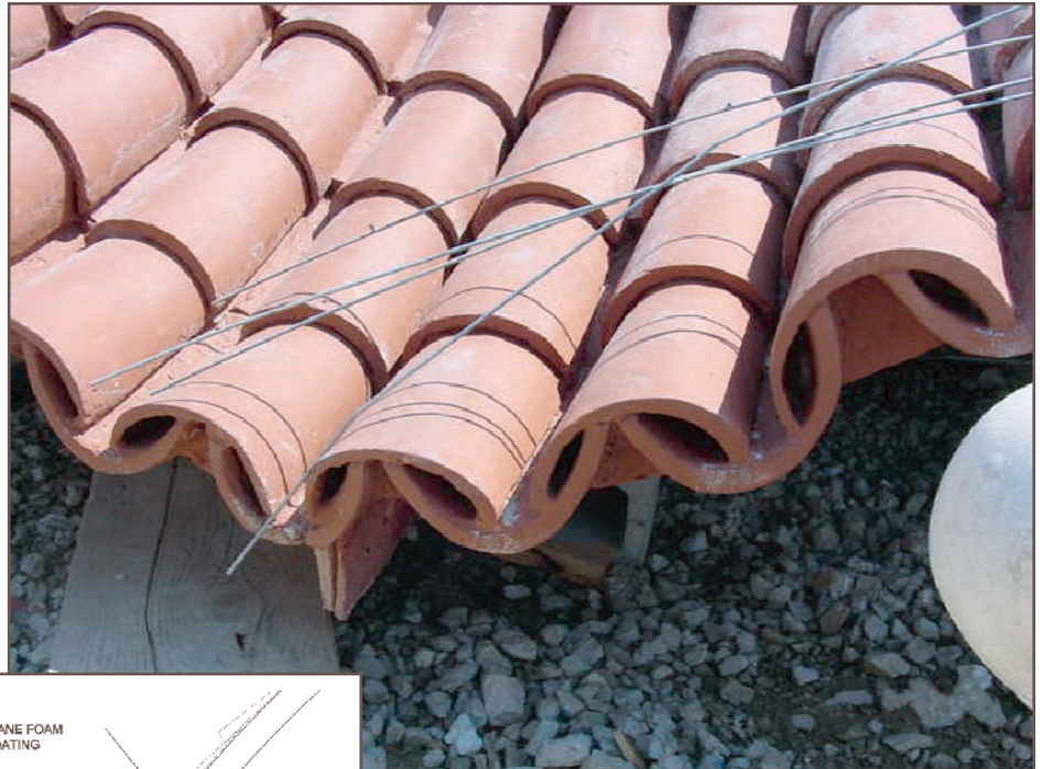
Above: Figure 6 - The crevices between the tiles were difficult to mold.
