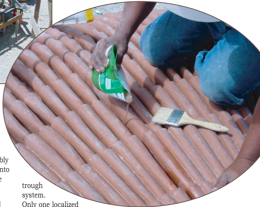
Below: Figure 10 - Sealing of the pie-shaped segment joints with pigmented resin.
