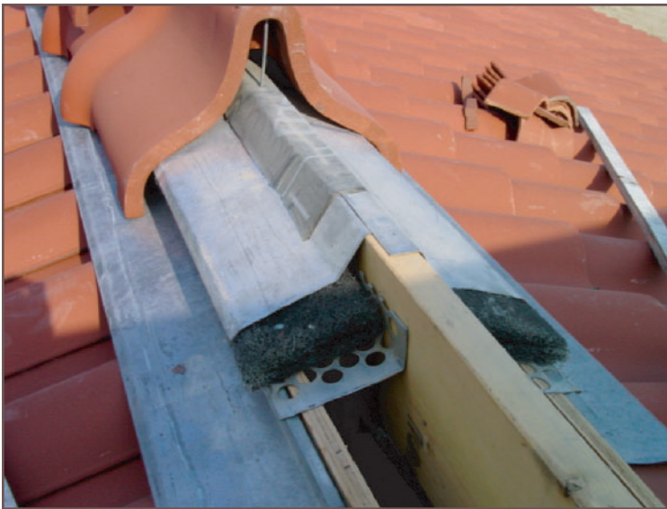
Figure 16 - Roof ridge configuration with ventilation provisions and a lightning arrest rod.
