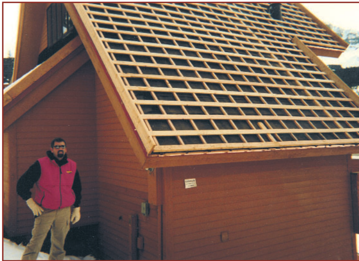
Above: New cold-roof system framework for concrete tile roof.
