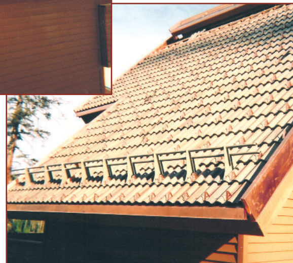
Right: New concrete tile roof with snow retention brackets.
