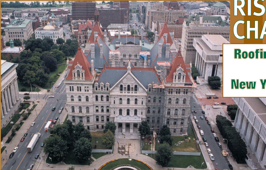
West facade of the NYS Capitol, Albany, NY, showing the roof project work area. The work platform at the eave of the corner tower (right side) is 185' above grade.
