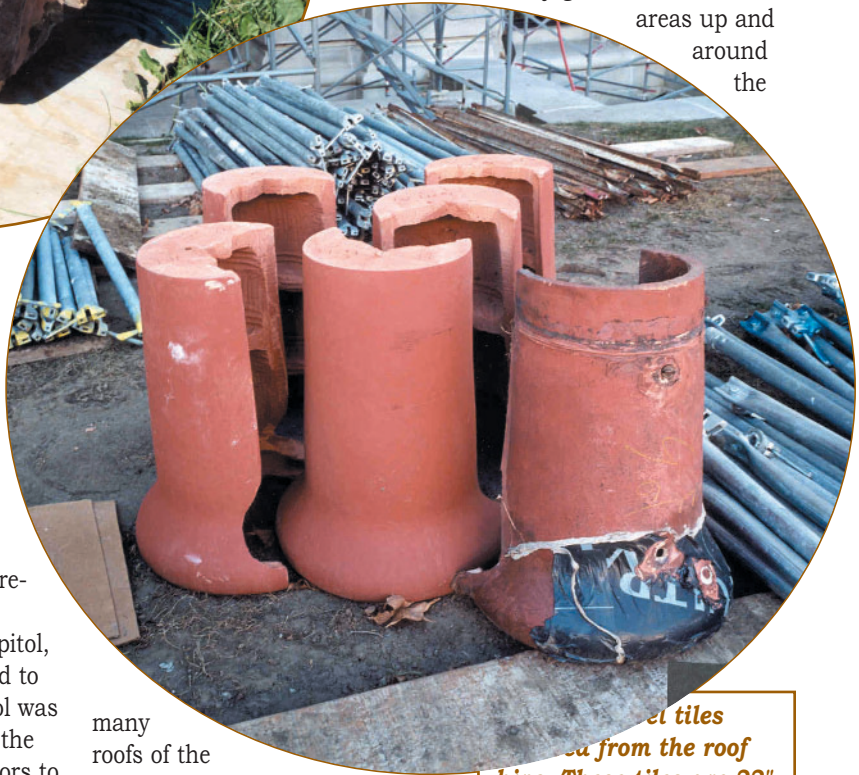
Existing ornamental terra cotta corner "ram's horn." This piece weighs 275 lbs. and is one of four corner pieces and four center sections that make up the base decoration of the large finials.
