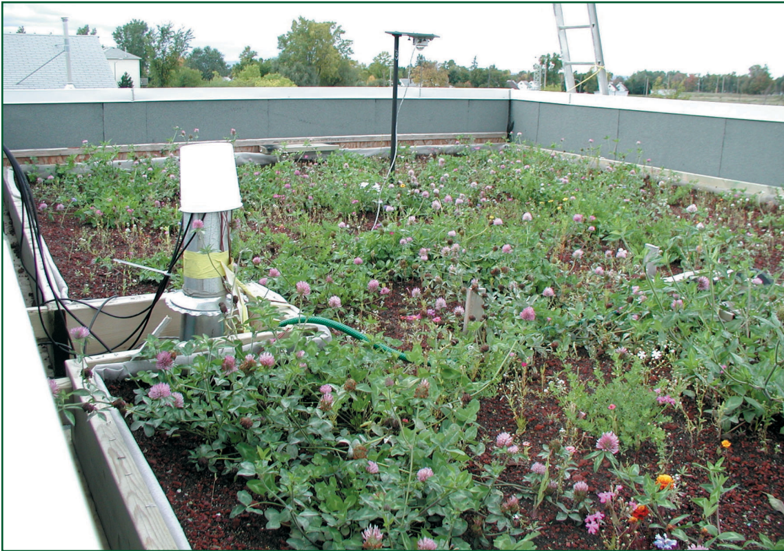
Figure 3 – A wildflower meadow (left) was established on the Field Roofing Facility (FRF) on the NRC campus in Ottawa (2001).
