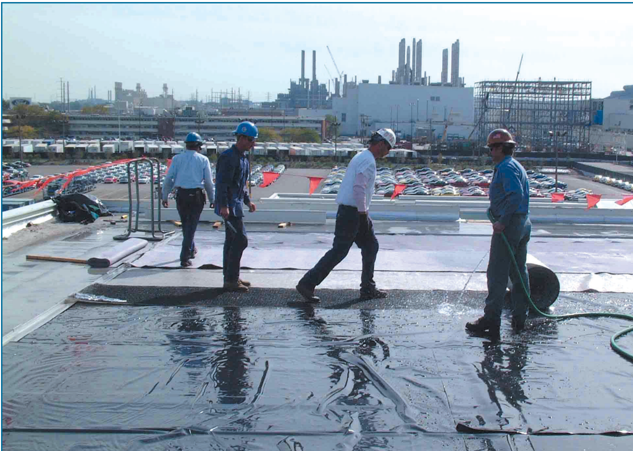
Figure 5: Green roof membrane application.
