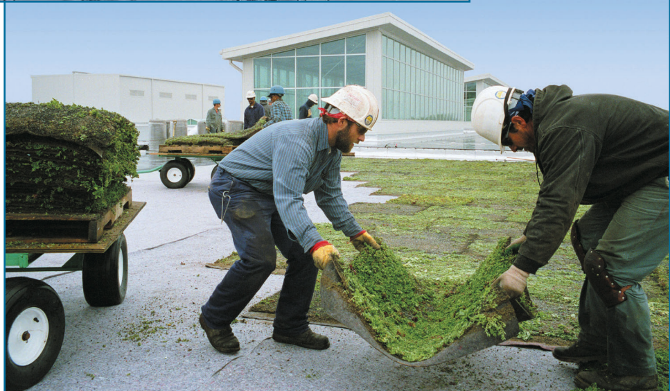
Figure 6: Workers position individual squares of sedum on fleece underlayment.
