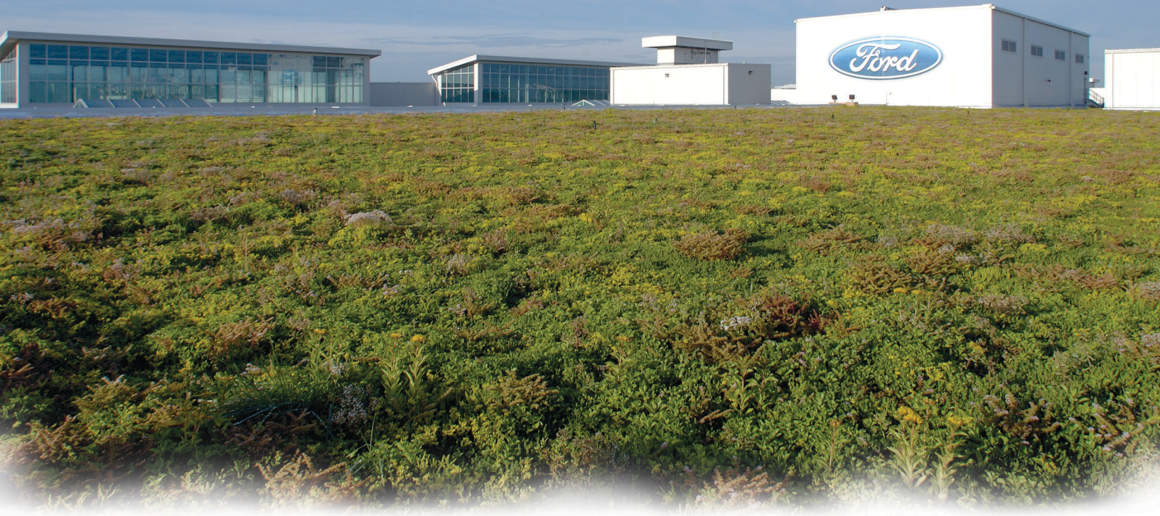
Figure 1: Ford roof in summer.
