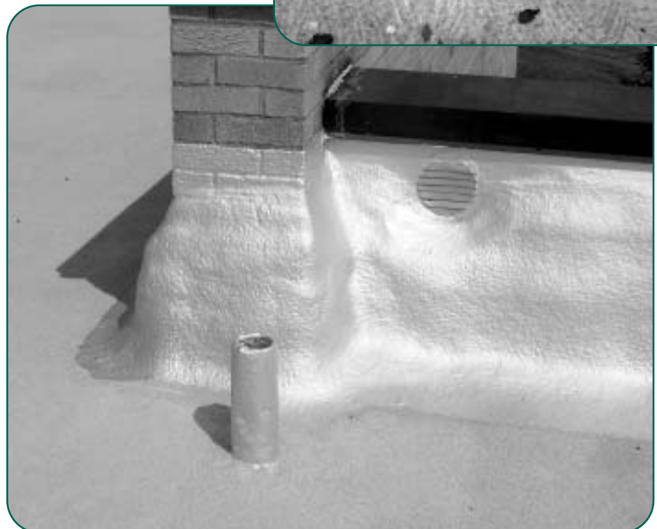
Figure 8 - SPF low wall flashing application.
