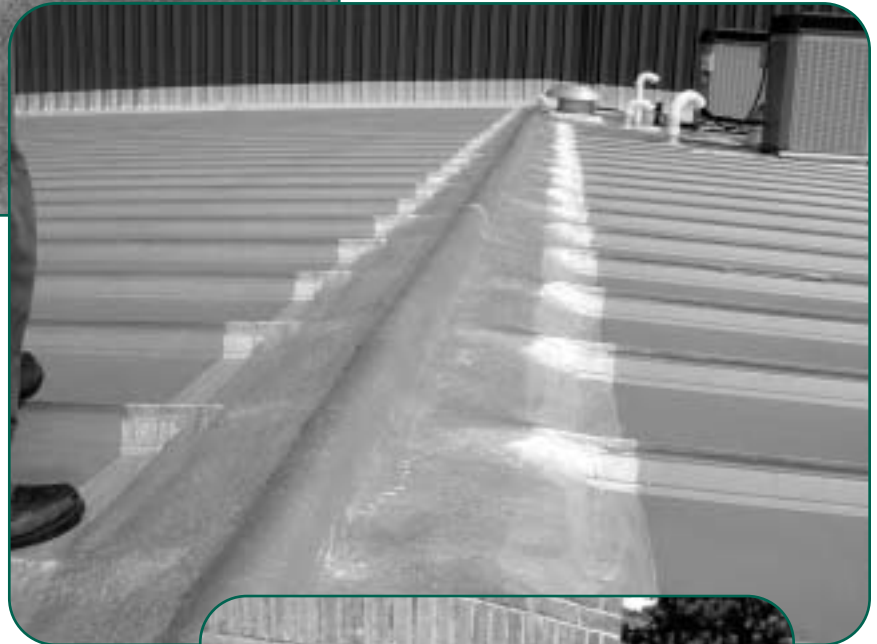
Below: Figure 2 - Metal roof expansion joint.
