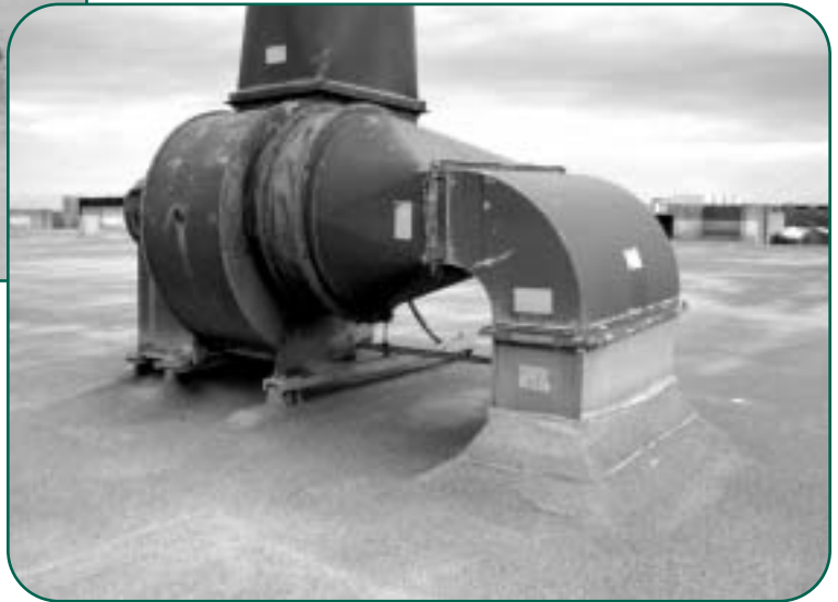
Figure 10 - Equipment support – low curb.
