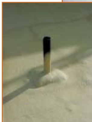
Left: SPF roofs are seamless and self-flashing for improved resistance to lifting and peeling failure during high wind events. The SPFA reports that SPF's wind uplift resistance exceeded the capacity of UL's equipment during testing.
