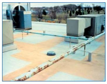
Roof mounted HVAC units should be raised and curbed, but typically don't require additional counterflashing.
