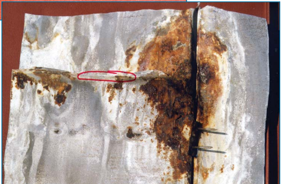
Right: Figure 9: View of the underside of the panel shown in Figure 8. The circle indicates the upper end of the down-slope panel. A panel clip with two nails occurs in the lower right portion of the photo.
