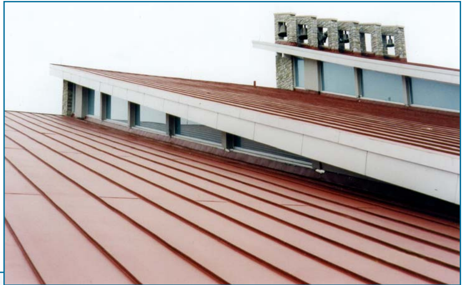
Figure 3: View of some of the clerestory windows. Although the roof overhangs provide some protection from rainfall, they do not protect the windows from wind-driven rain.
