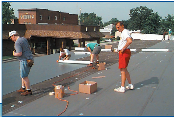
Church members assisted in the installation of the roof systems.
