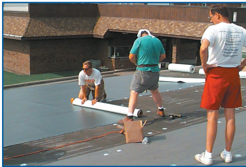
Peter Garrigus of Trufast (formerly of Stevens Roofing) and Dave Scott roll out TPO sheets.
