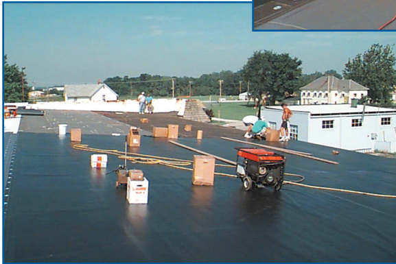
Installing black TPO sheets on east side of church roof.
