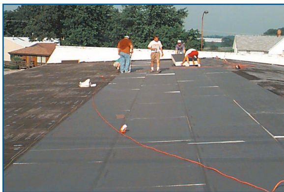
Layout of "cool black" TPO sheets on west side of church roof.
