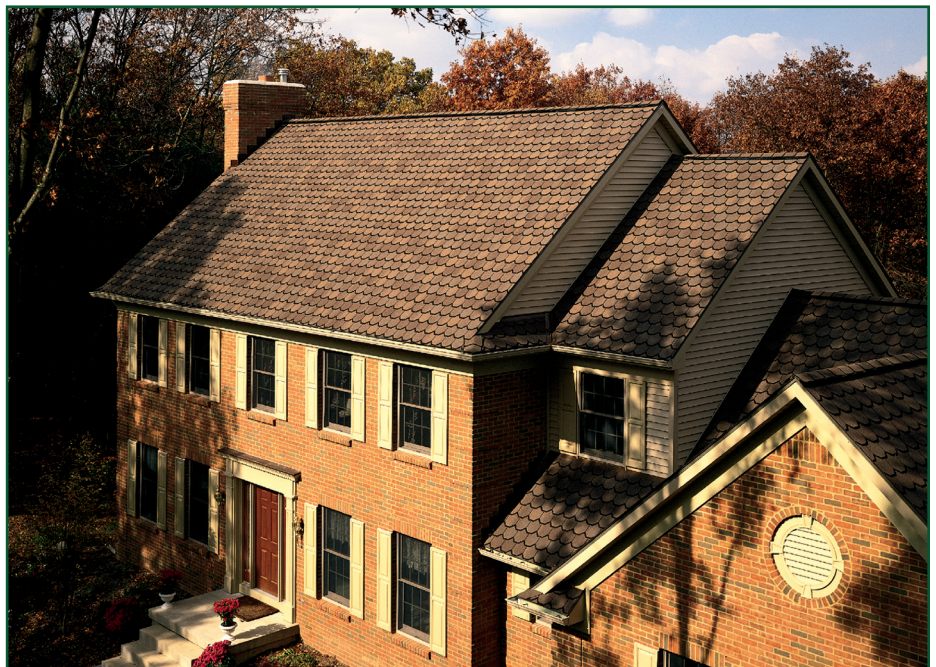
Removing heat and moisture from the attic with a proper ridge vent system is fundamental to maintaining a healthy roof structure.
