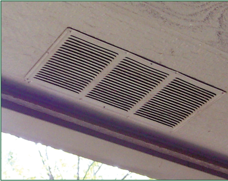
To work effectively, exhaust vents need proper intake ventilation at the soffit or undereave, like the rectangular undereave vent pictured here. Intake and exhaust vents work together to form a balanced attic ventilation system.
