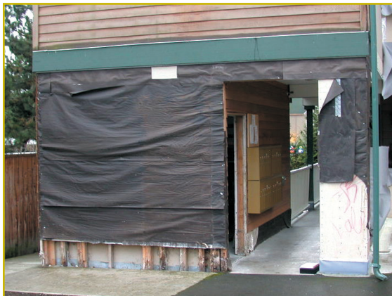
Photo 1 - Overview of the work area.
