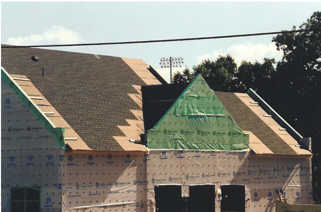
Figure 3 and 4: The photo at left shows racked shingles. The one below shows the correct way to lay shingles.
