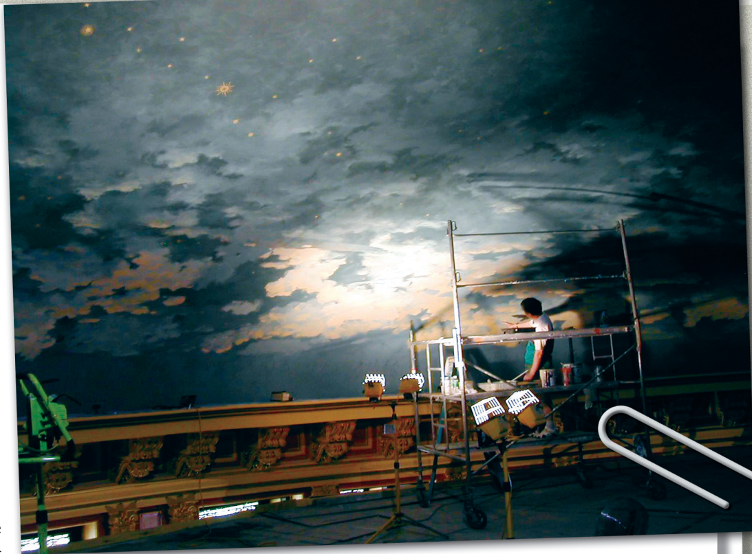
The stars were mapped onto the floor using a laser so their placement could be accurately recorded. They were then remapped onto the ceiling and painted.
