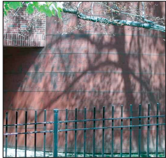
Figures 9 and 10: Only the initial aesthetics are affected by this natural but unusual weathering. With time, the copper should take on a uniform brown, bronze, and eventually blue-green color of natural patina.
