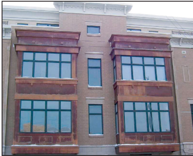
Figures 9 and 10: Only the initial aesthetics are affected by this natural but unusual weathering. With time, the copper should take on a uniform brown, bronze, and eventually blue-green color of natural patina.
