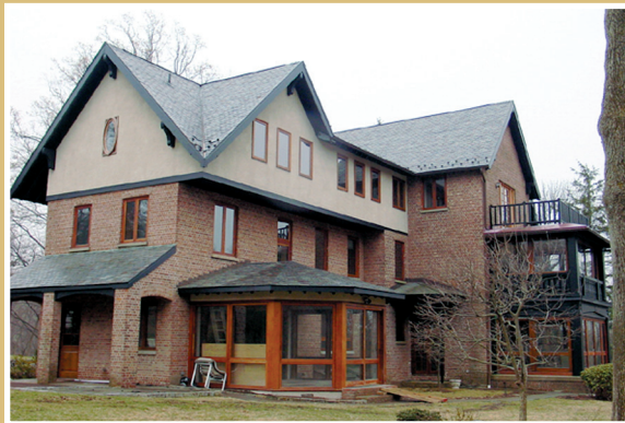
Ten-year-old slate roof on a private residence condemned by roofing contractors. The nominal snow guard damage, however, was covered by homeowner's insurance; the roof did not need to be replaced at all. (Photo by Joseph Jenkins.)
