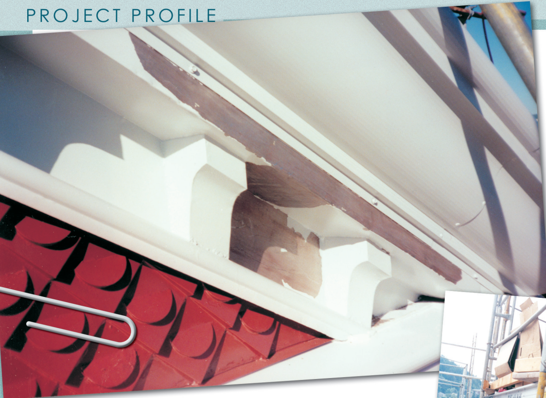
Below: The existing paint finishes were lead-based, requiring the use of polyethylene sheeting to catch and allow for the proper disposal of the removed paint.
