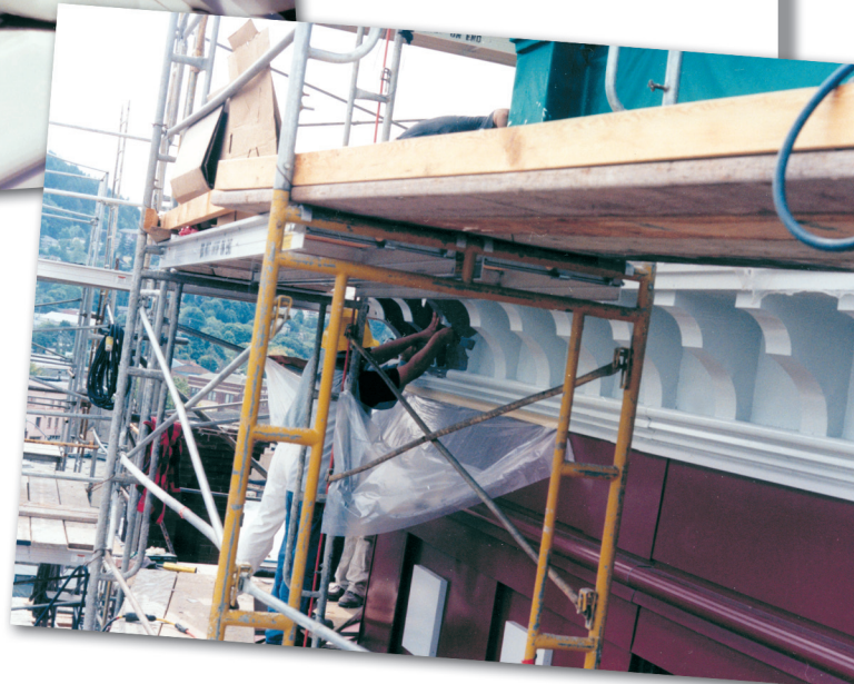
Below: The existing paint finishes were lead-based, requiring the use of polyethylene sheeting to catch and allow for the proper disposal of the removed paint.
