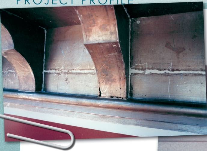
Left: Where paint removal revealed deteriorated metal where decorative sheet metal had been intended for retention, the sheet metal was repaired in situ.
