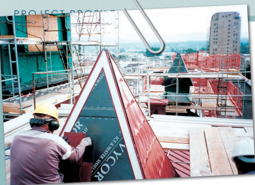
The foreground cupola is being shingled, while the background cupola has only the self-adhering waterproofing underlayment in place and breathable underlayment is being installed at the central clock tower.
