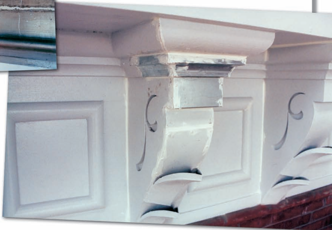
Below: A typical in situ repair of a retained corbel at the main building cornice.
