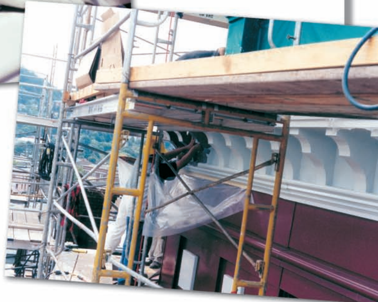
Below: The existing paint finishes were lead-based, requiring the use of polyethylene sheeting to catch and allow for the proper disposal of the removed paint.
