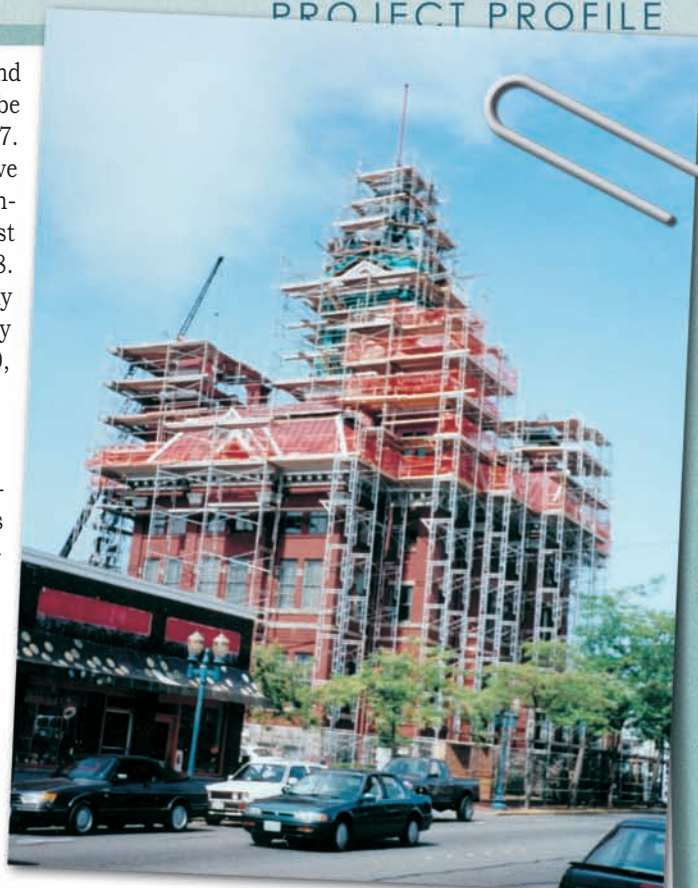
Although some work on the building envelope occurred below the roof line at the main building cornice, full scaffolding was erected, primarily for the replacement of the roof.
