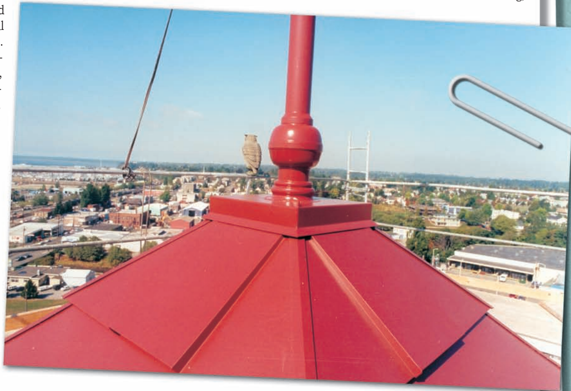
A particular highlight of the work was the completion of the uppermost Bermuda-style roof with its raised central panels that caps the central clock tower.
