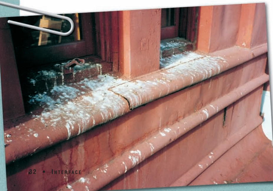
This detail view of the metal cladding at the southeast corner cupola clearly revealed the failed seams, multiple small repairs (some of which had also failed), and the accumulated bird excrement to be dealt with.
