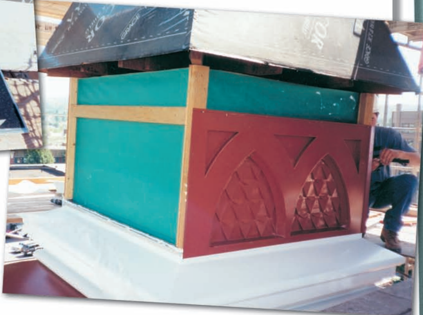
Right: "Fish scale" panels are being reinstalled at the northeast cupola with new wood blocking at panel perimeters. Note the use of breathable underlayment at the cupola wall and waterproofing underlayment at the pyramidal hipped roof above.
