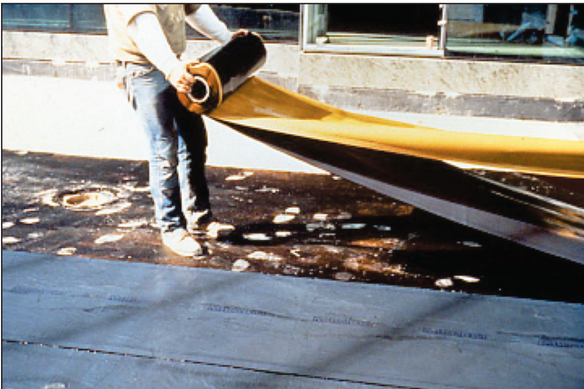
Figure 5: Self-adhering rubberized asphalt sheet membrane.
