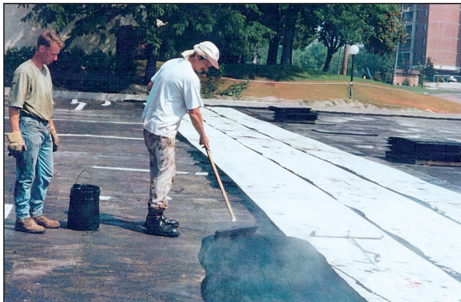
Figure 8: Hot-applied liquid membrane (American Hydrotech)
