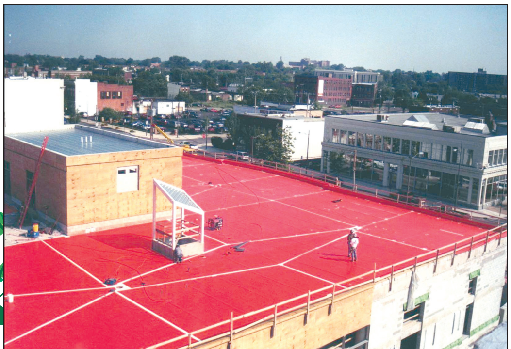
Figure 10: Compartmenting of loose-laid PVC membrane (Sarnafil)
