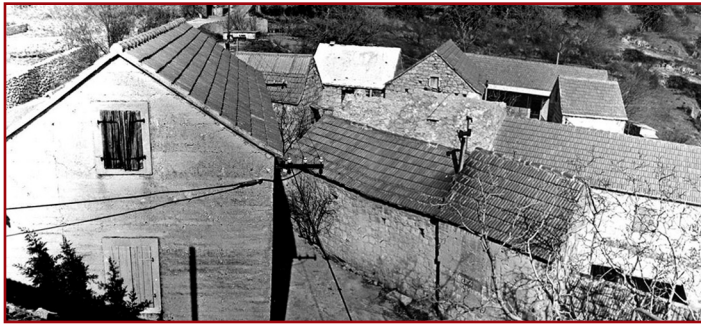
Figure 1: Neighboring stone and clay tile roofs common to the area.
