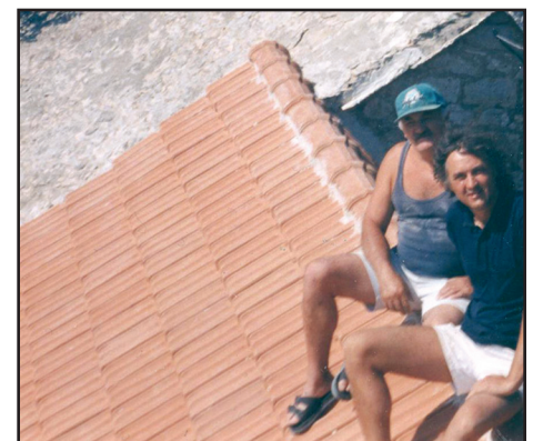
Figures 8: The roof is finished, but....!
