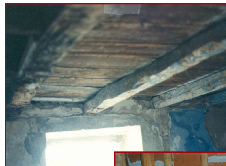
Figures 10a and 10b: Corrective attempts from inside; attic boards and joists were later removed.
