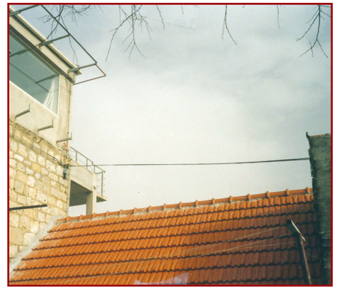
Figure 14: The roof repair is finally done properly.
