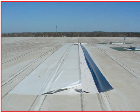
Photo 6: Membrane slit by a tumbling exhaust unit.
