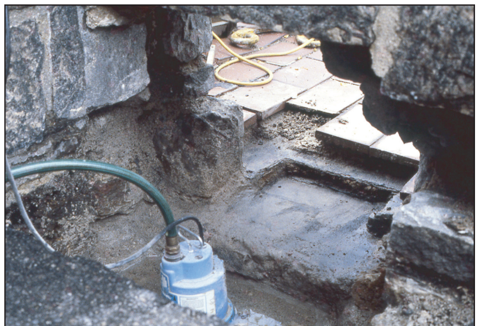
Figure 1: Exposing membrane for repair.
