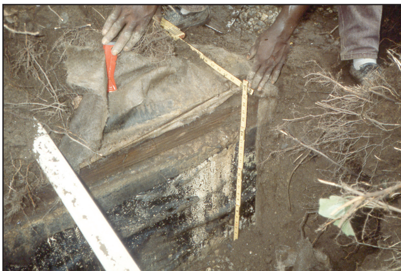
Figure 2: Root intrusion.
