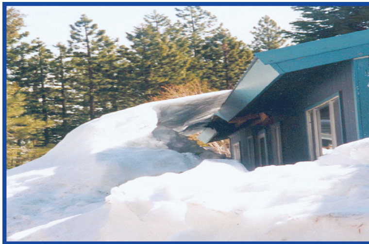
Photo 2: Dormers can be torn off.
