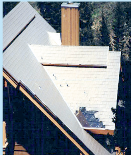
Photo 1: Damage to flat seam metal roofing.
