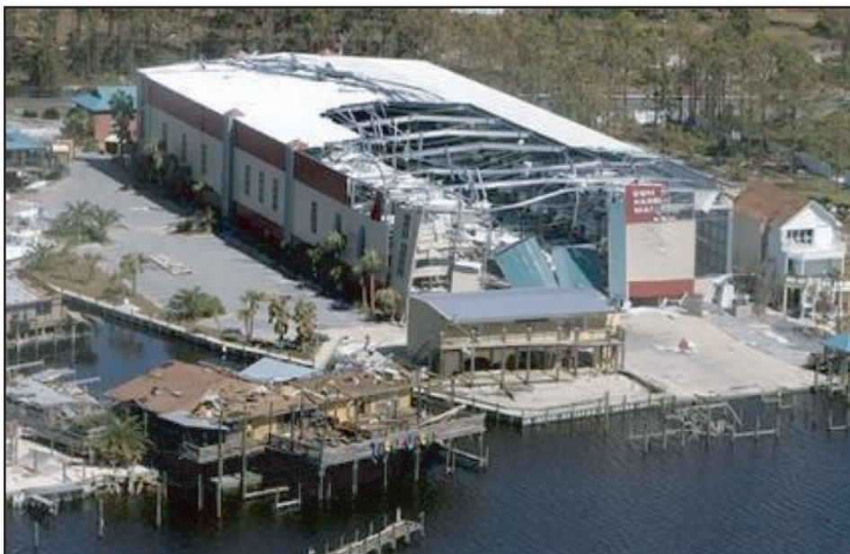
Figure 6: Damage caused by Hurricane Ivan on the Florida panhandle. This structure appears to have a large damaged door opening facing the water. The structure would likely be considered "partially enclosed."
