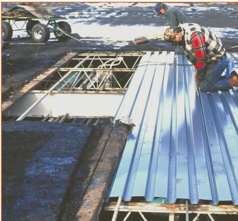
Portions of this steel roof deck are being replaced.
