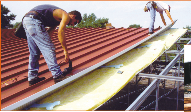
Flat roof being retrofitted with a sloped standing seam metal roof.
