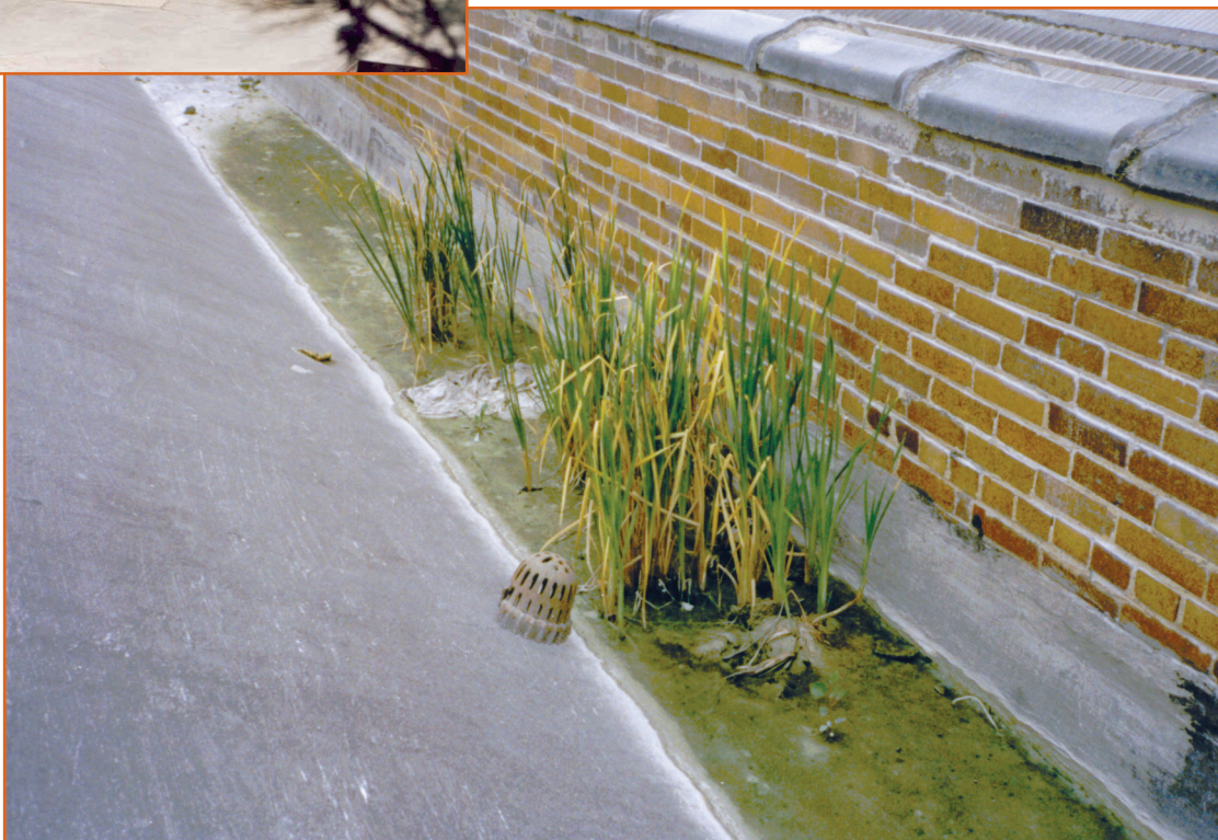
This roof drain is blocked with plant growth and sediment.
