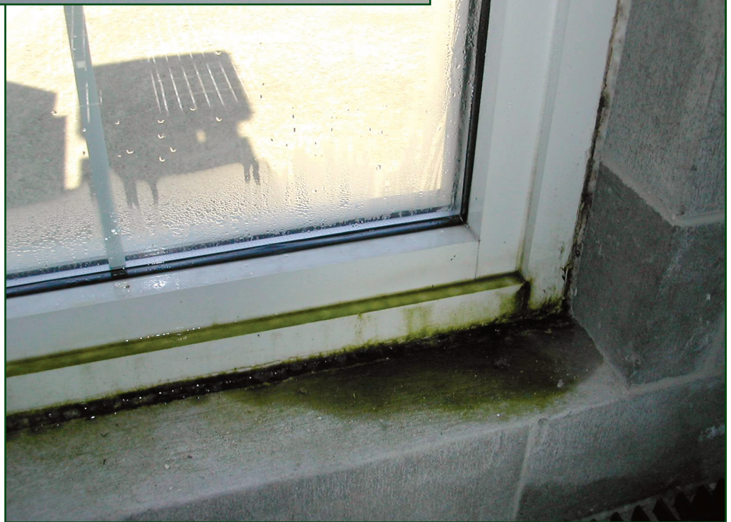
Below: Photo 3 – Failure to provide sufficient condensation resistance on fenestration in high humidity spaces can lead to problems ranging from mold growth on interior surfaces to premature failure of the product.
