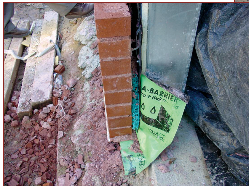
Photo 3: Narrow wall cavity difficult to keep clean during construction.
