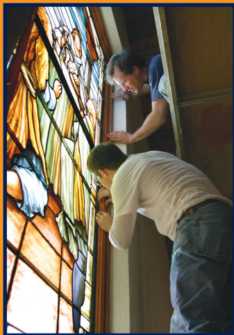
Finish trim is reinstalled after the window is in. The dark bar in the center is the T-bar, which was added.
