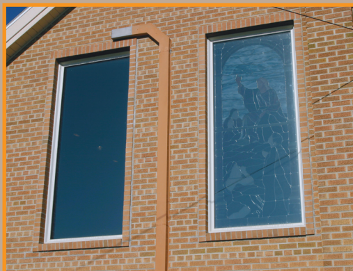
The exterior glazing remained intact through the stained glass installation.
