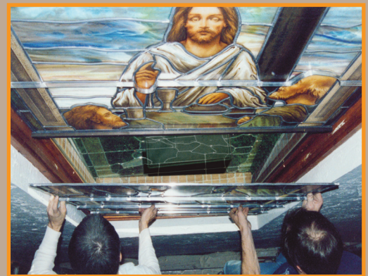
Each panel is secured separately. Small ventilation screens or "breathers" have been inserted into the frame to release heat and moisture from between the existing and new glazings.
