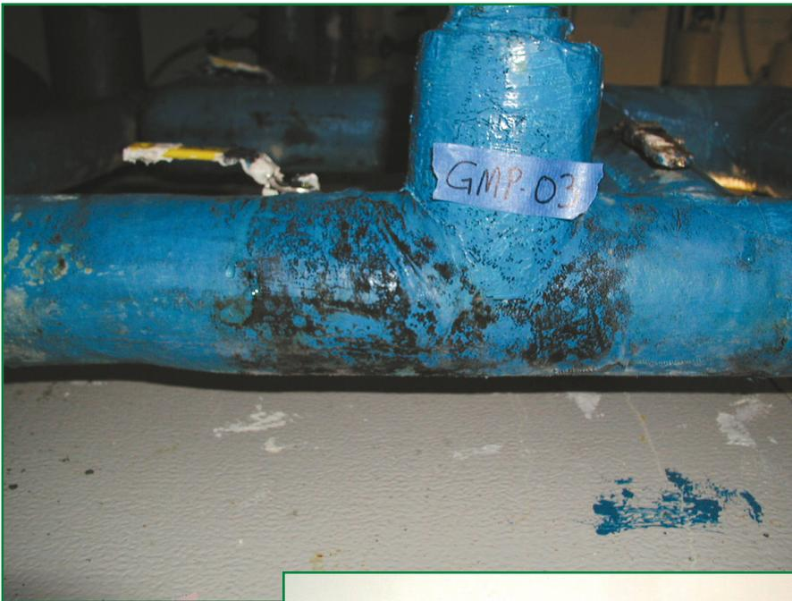
*Photo 8: Mold on asbestos-containing pipe insulation.*
