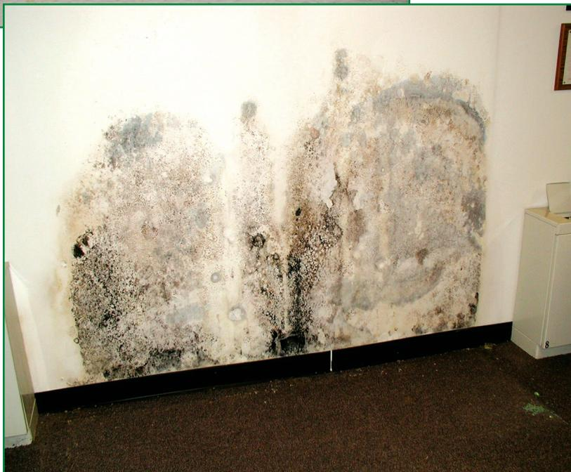
*Photo 9: Mold on gypsum wallboard with asbestos-containing joint compound.*
