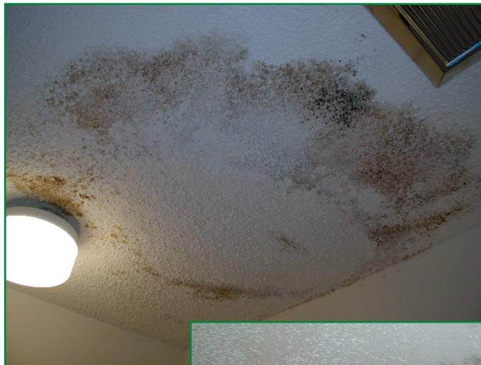
*Photo 1. Mold growing on asbestos and lead-based paint.*
