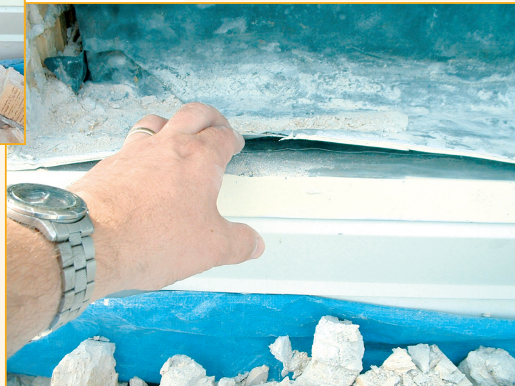
Photos 1 and 2. Remedial through-wall masonry flashing repairs are often expensive and disruptive to an owner's operations. Roof consultants routinely investigate and specify transitions between systems, such as roofing and masonry.
